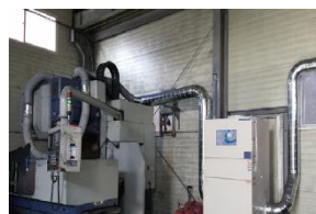
Dust collection from drilling operations
